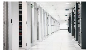
Security and environmental monitoring system
